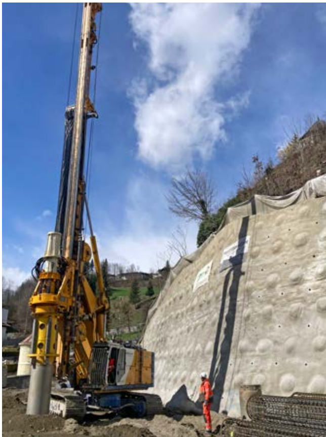
EXECUTION OF LARGE DIAMETER BORED PILES
