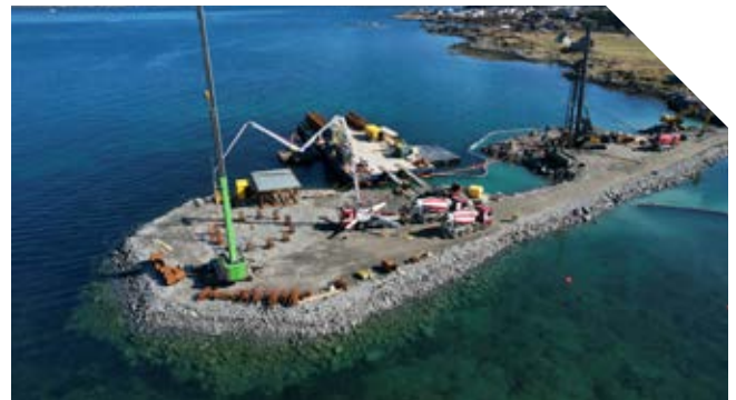
CONCRETING AXIS 4 AND DRILLING WORK ON AXIS 3
