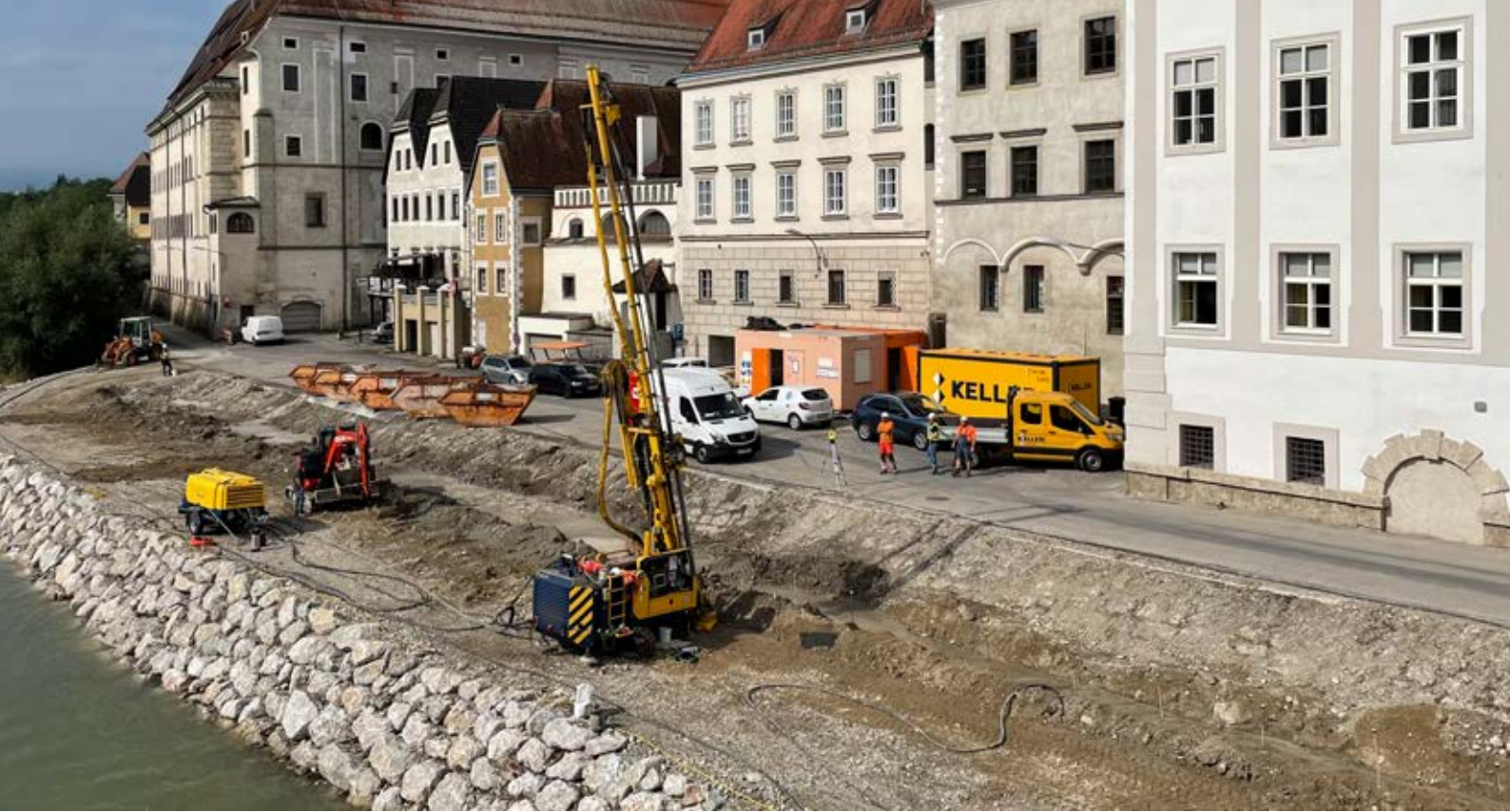
ENNSKAI CONSTRUCTIONS SITE, STEYR
