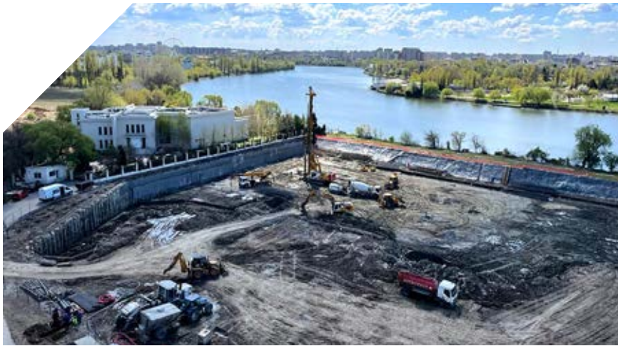
PHOTO DURING THE FOUNDATION PILES EXECUTION
