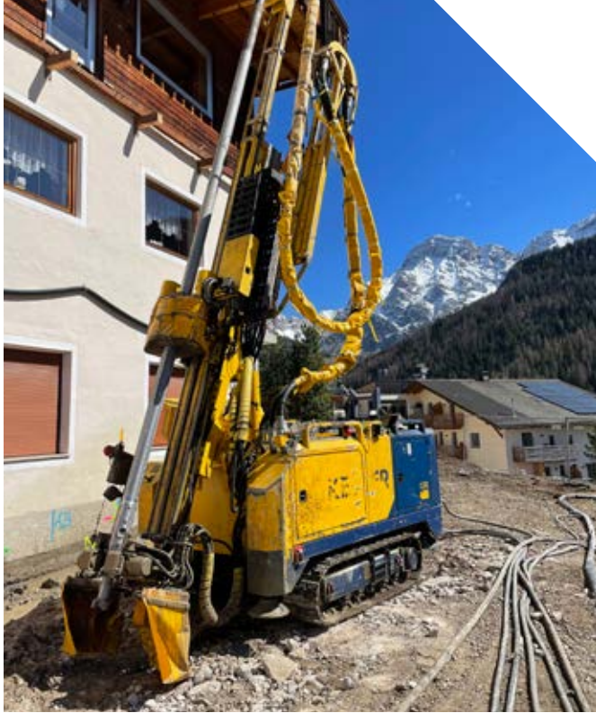
HOTEL EXTENSION – UNDERPINNING WITH JET GROUTING Hotel Alpenrose – Wengen
